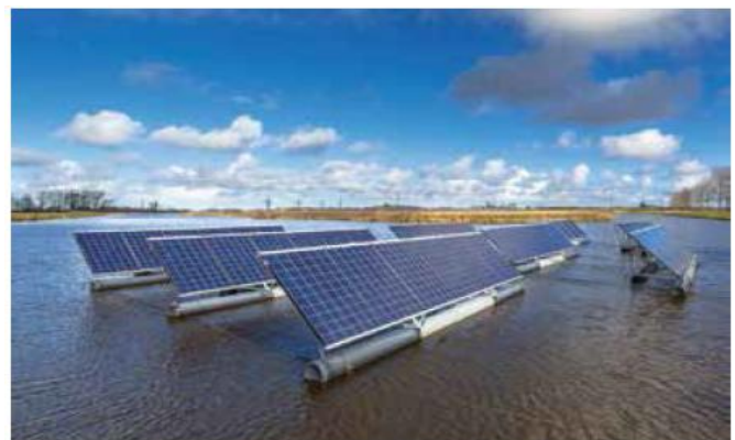
Figure 14: Floaters design
