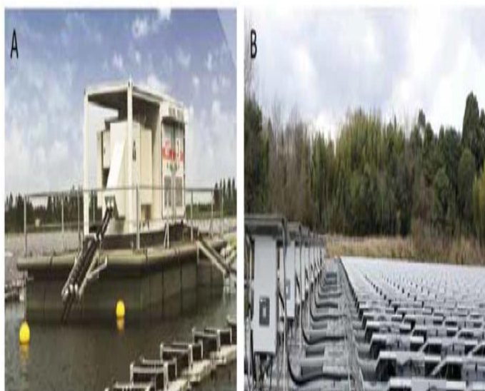
Figure 10: (A)Central inverter placed on floating platform at China. (B) String inverter
